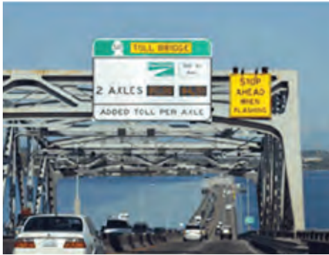
State Route 520 Bridge
